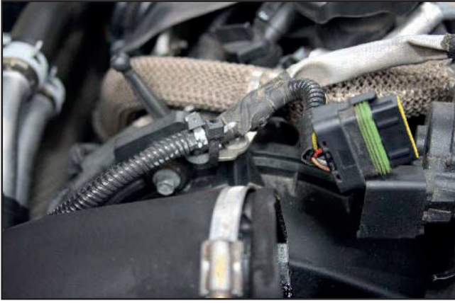
Tie-wraps – right hand EGR pipe bracket
